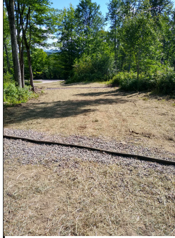
↑ Water bars on sloping road Jillian moving straw blower →
